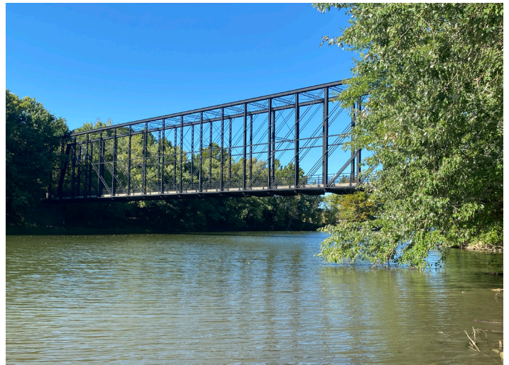
The Triple Whipple bridge, now a pedestrian walkway, sits just off Indiana State Route 56 in Dearborn County, south of Aurora.
